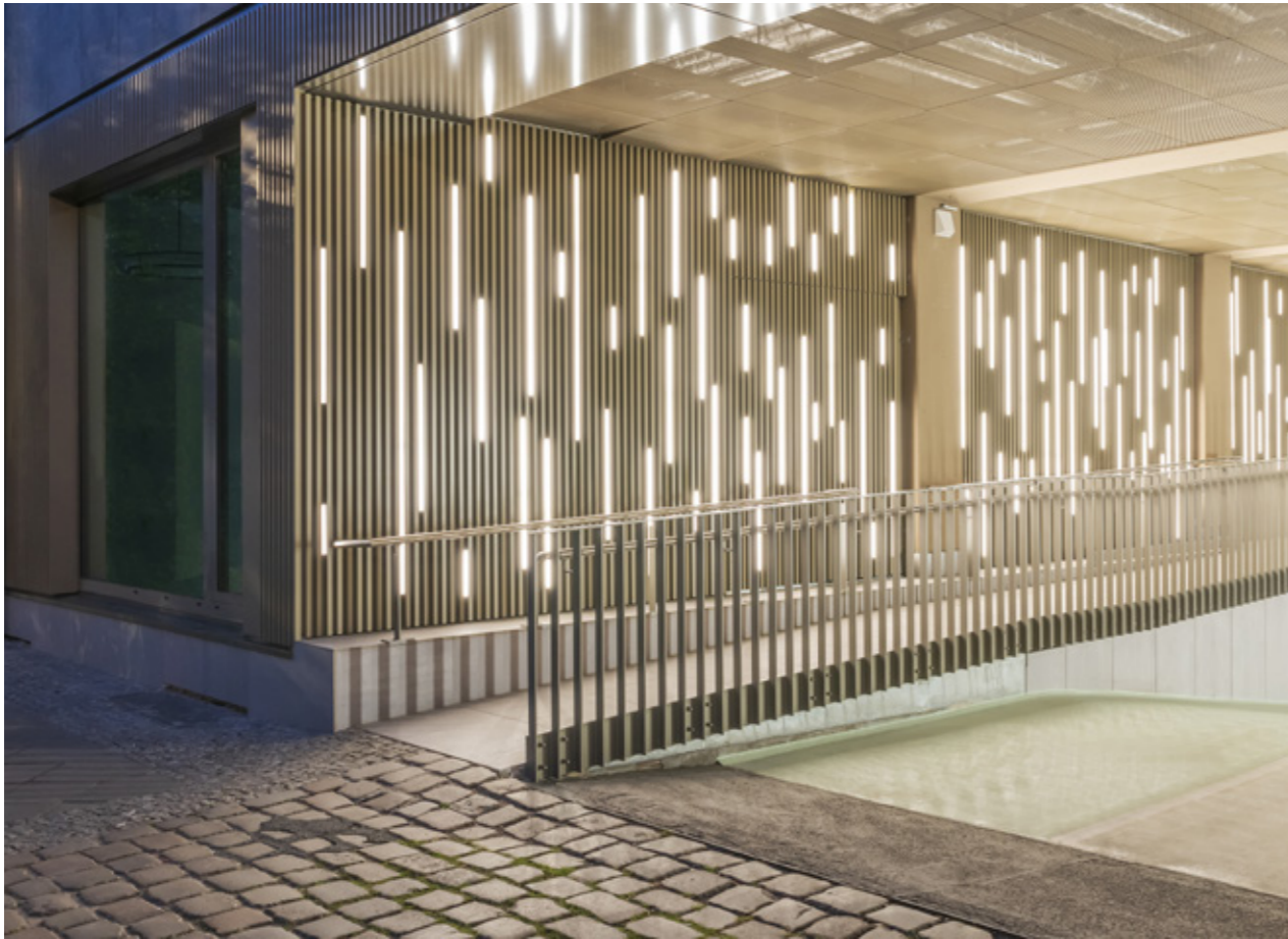
LED strips bring your façade to life in the evening. The IP67 LEDs are dimmable, available in warm white light and made to measure. Application possible in combination with all Linarte profiles.
